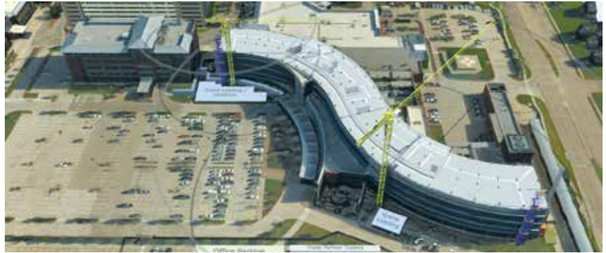
The picture above is a rendering for the expansion. Once the new parking garage is complete, work will begin on two new hospital floors and a ninth operating room.
